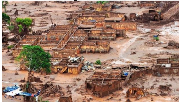
Figure 1 – View of the Bento Rodrigues district after the Fundão dam collapse.
